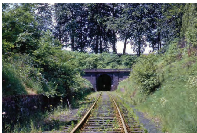
The now buried east portal in June 1965. Photo Bill Wright
